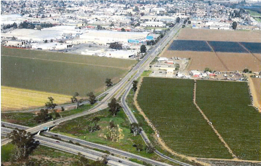
This aerial photograph shows where Riverside Drive merges with Highway 1 in Watsonville. — Tarmo Hannula/The Pajaronian file
