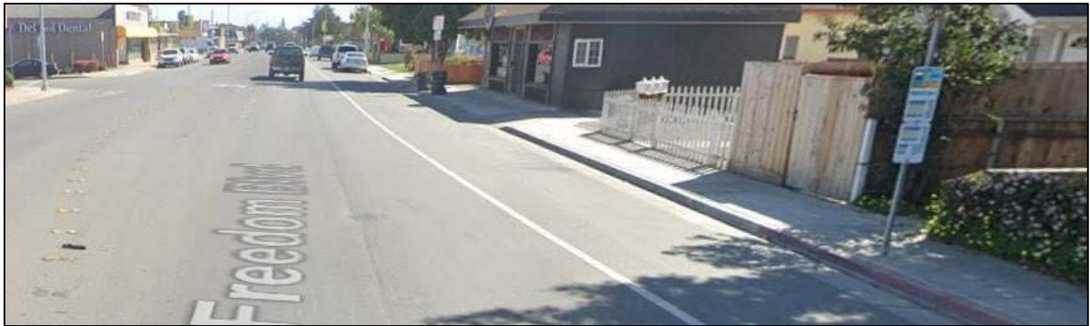
Bus stop located more than 100 feet from an existing crosswalk at 1115 Freedom Boulevard, Watsonville, CA
