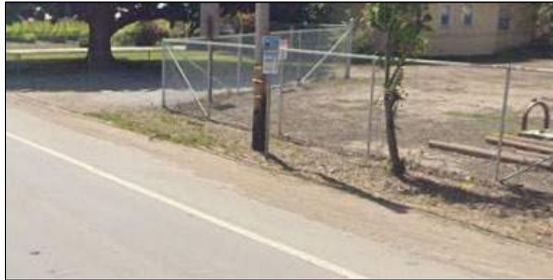
Bus stop lacking sidewalk, a concrete pedestrian waiting area, and an ADA path of travel at 2838 Freedom Boulevard, Watsonville, CA
