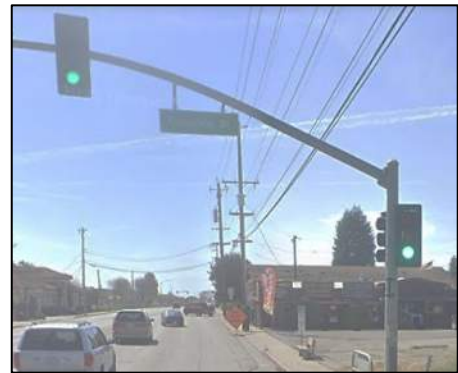
Bus Stop Located Far-side of an Intersection at 217 Green Valley Road, Watsonville, CA
