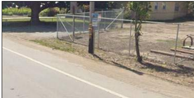
Bus stop lacking sidewalk, a concrete pedestrian waiting area, and an ADA path of travel at 2838 Freedom Boulevard, Watsonville, CA
