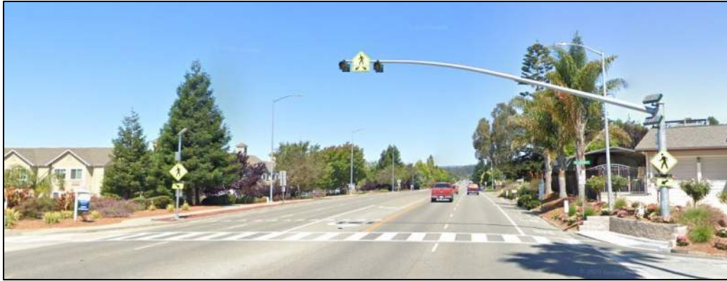
Bus Stop Near a Pedestrian Hybrid Beacon (PHB) at 7470 Soquel Dr, Aptos, CA
